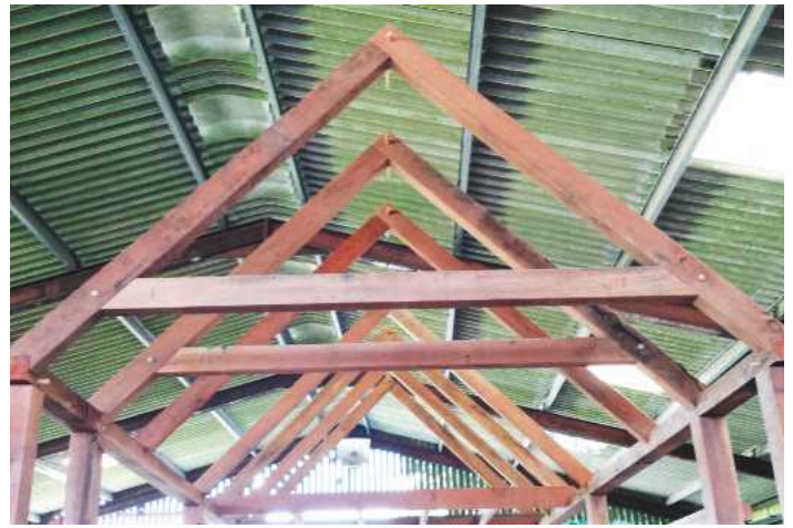
Pegs, as seen in the roof trusses, hold the frame together
